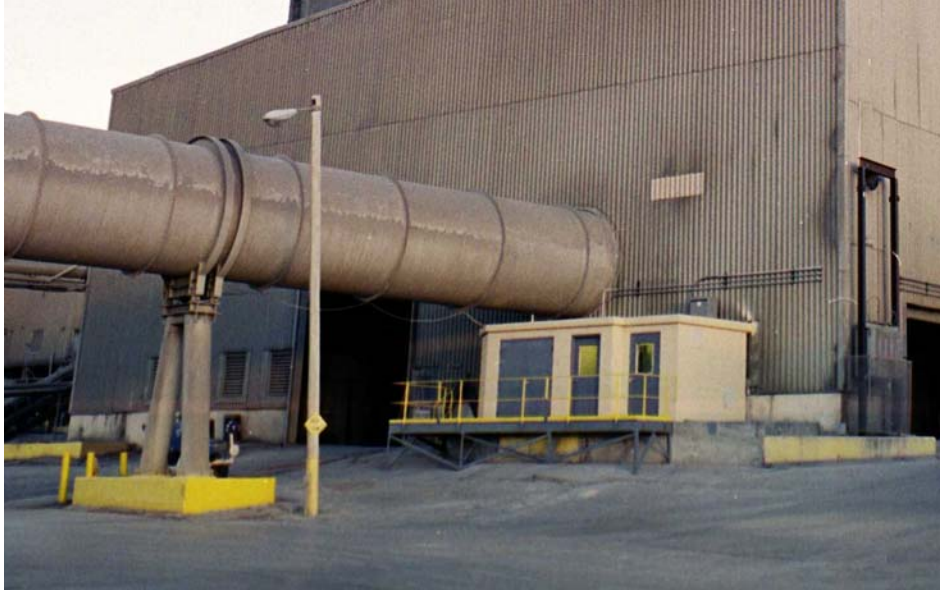
Figure 2. XRD room next to mill building at Leamington
